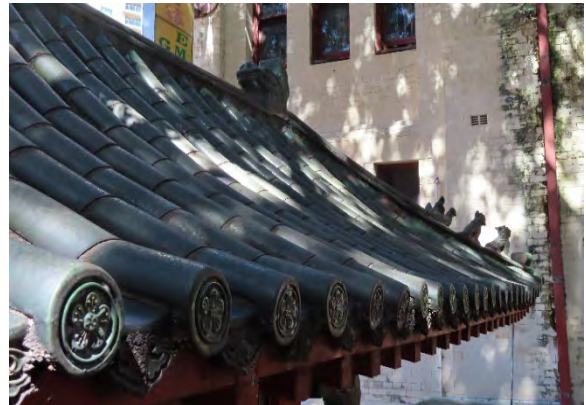
Figure 4.42 Tiles of the western side of roof.
