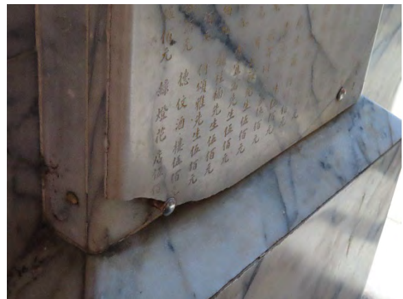
Figure 4.25 Chipped marble plaque.
