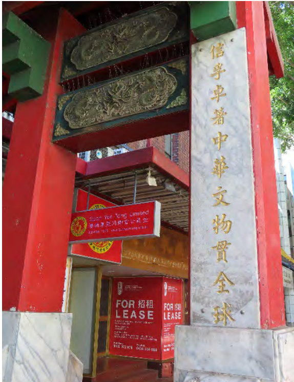
Figure 4.12 Gateway marbles plaques fixed to the reinforced concrete frame on the eastern bay.
