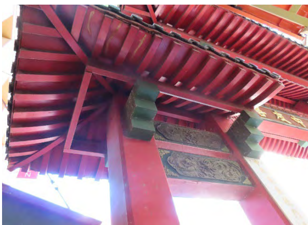
Figure 4.34 View of curved rafters and exposed roof structure of lower roof.
